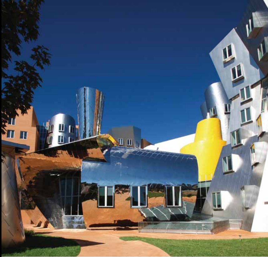
The site design at the Ray and Maria Stata Center at Massachusetts Institute of Technology, Cambridge, is a good example of sustainable site systems design.
